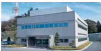
Shikoku Operations Lab Center
