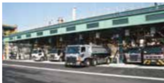
Shikoku Operations Lorry loading facilities
